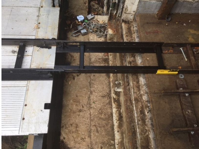
CARRIAGE STORE TO PLATFORM ROUTE VIA THE ATTACHED HINGED LINK RAIL
